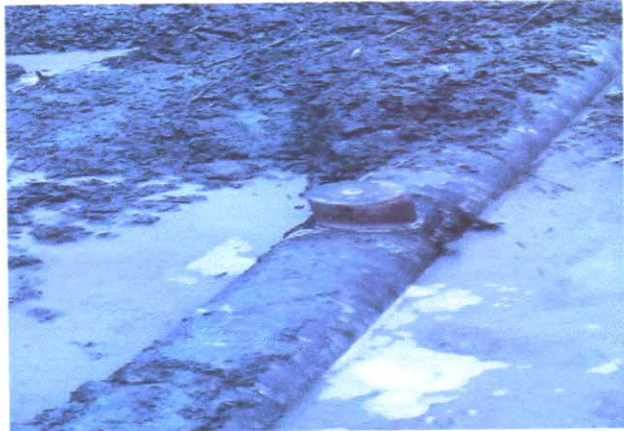
Figure 2: Coned after repair on the Pipeline .
